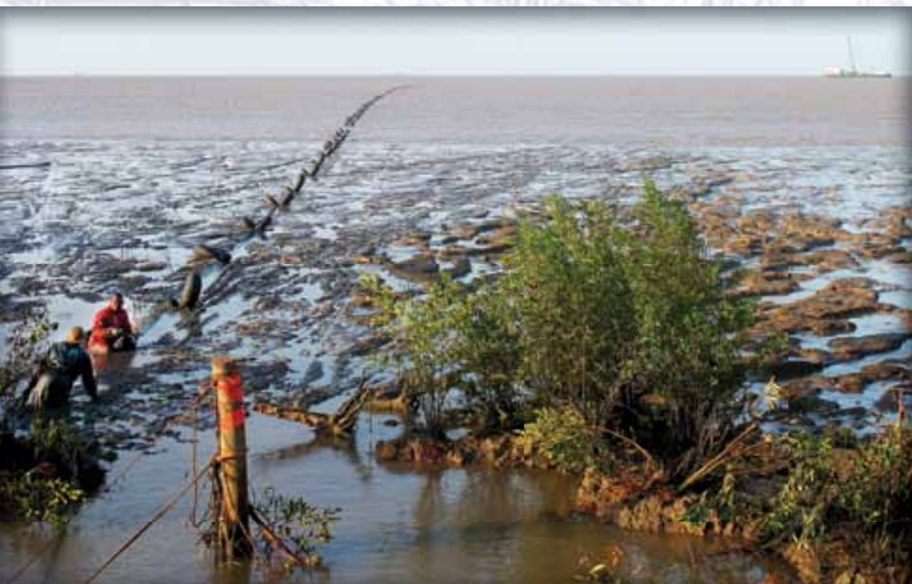
SG-SCS Zeekabel Pre-shore landing activiteiten.
